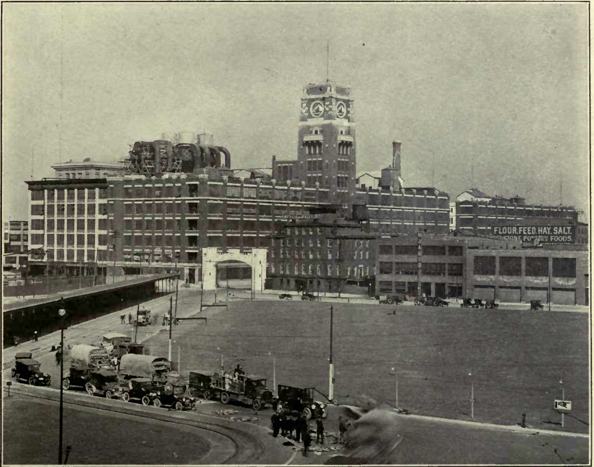
Victor Talking Machine Co., Camden, N. J. Ballinger & Perrot, Architects. Irwin & Leighton General Contractors This building is located near the Delaware River, the basement of the working establishment being some five or six feet below high tide. Foundation work waterproofed with Truscon Waterproofing Paste, Concentrated .
